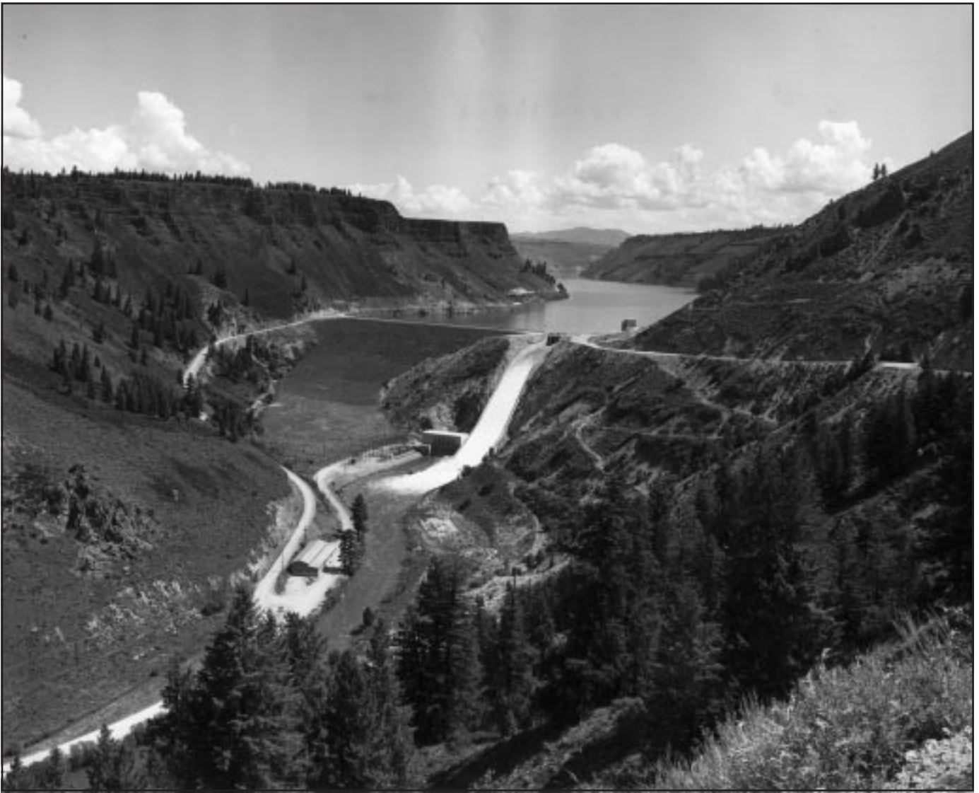
Boise Project, Arrowrock Division, Anderson Ranch Dam. Located on the South Fork of the Boise River, 20 miles northeast of Mountain Home, this earthfill structure is 456 feet high and has a storage capacity of 493,200 acre-feet.
