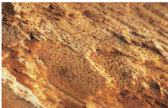
Figure 128. Decay from laminated root rot has distinctive round pits about pinhead-size.
