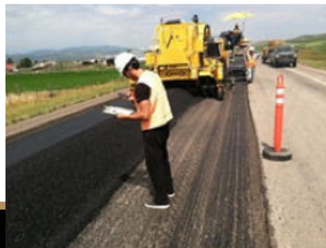
PhD student Ahmed Muftah checks the mix temperature during construction of the fiber project on US-30
