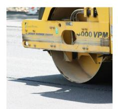
1<sup>st</sup> pass entire drum on hot mat with roller edge off joint approx. 6-12"
