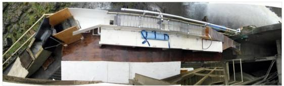
Figure 1. Overhead view of the Denil and trap used to collect adult steelhead and Chinook salmon at Willamette Falls Dam in 2012.
