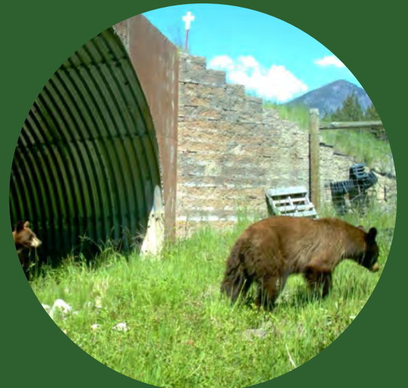
Figure 2.21 Example of a wildlife underpass
