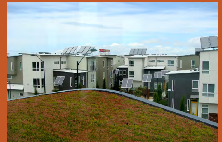
Figure 2.31 View of green roof and solar panels.
