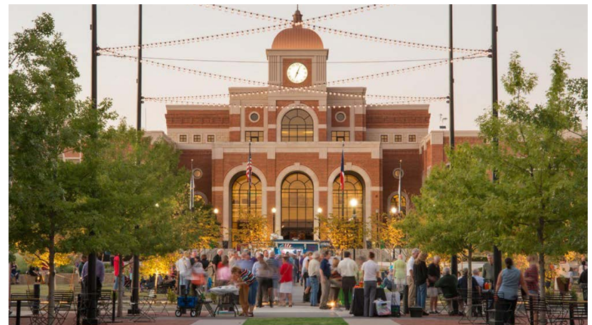
Lewisville's Wayne Ferguson Plaza. Image courtesy of Design Workshop
