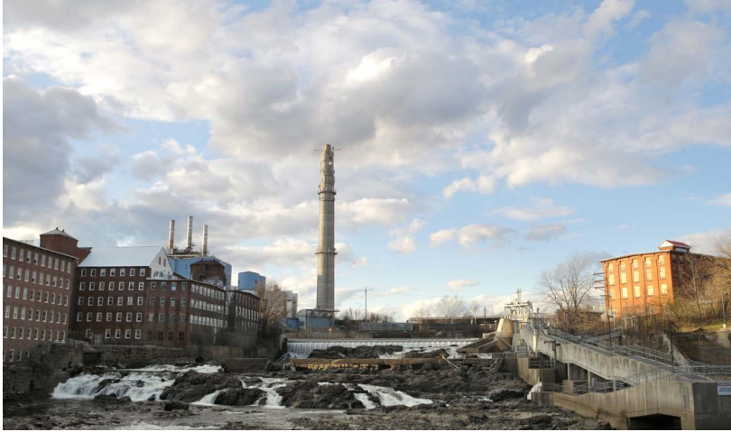
Biddeford, Maine's trash incinerator, pre-demolition. Image courtesy of Portland Press Herald
