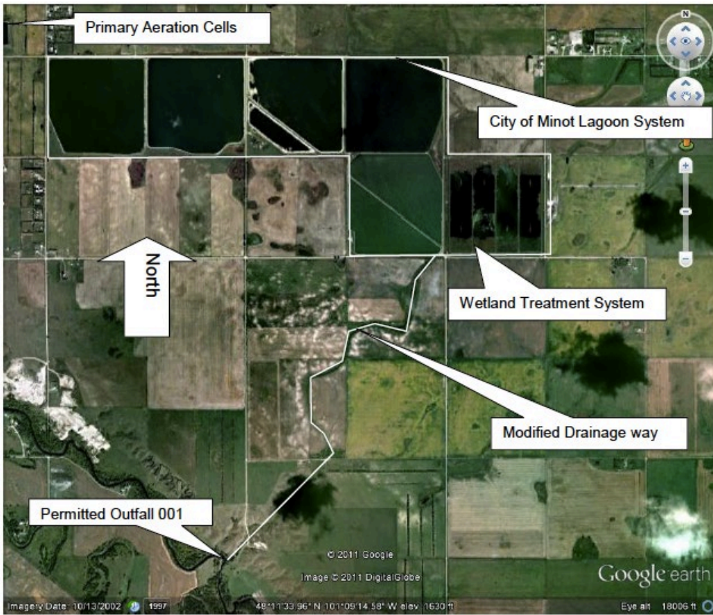
Figure 16. Aerial map of Minot, North Dakota, wastewater treatment works. Google Earth, 2018.
