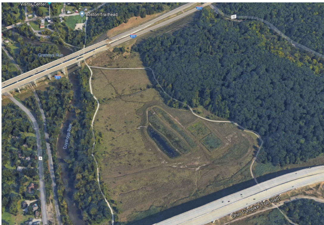
Figure 19. Aerial image of Boston Mills wastewater treatment wetlands. Google Earth, 2018.
