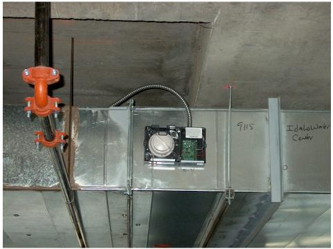
Typical duct mounted smoke detector Pic A12
