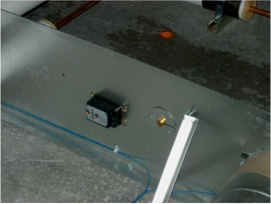
Typical installation of Temperature and Pressure Sensor Pic A9
