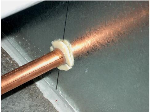
Typical pipe sealing through underfloor air plenum divider Pic A6
