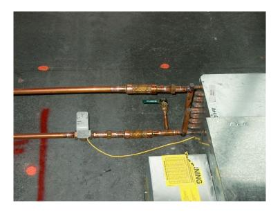
Typical fan box coil piping connection 02 Pic A4
