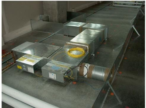
Typical Exterior Fan Box Installation Pic Al
