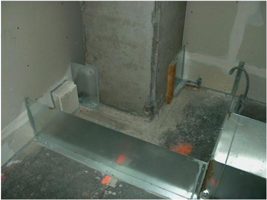
Typical Exterior Return Air Plenum Installation Pic A2
