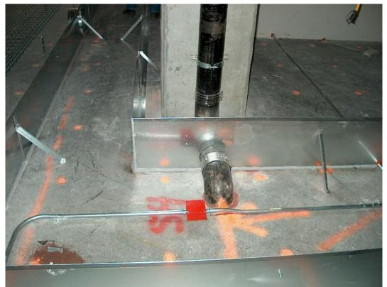
Typical RWL through underfloor air plenum divider Pic A7
