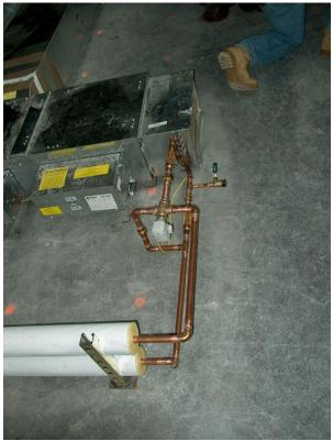
Typical fan box coil piping connection 01 Pic A3
