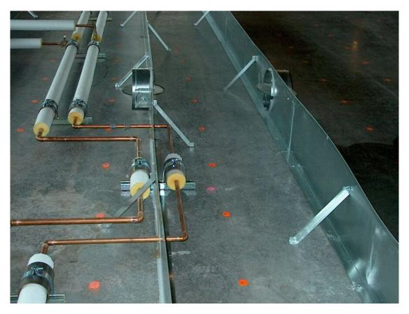
Typical fan under floor piping and supply air chase ways  $$\rm Pic\ A5$$
