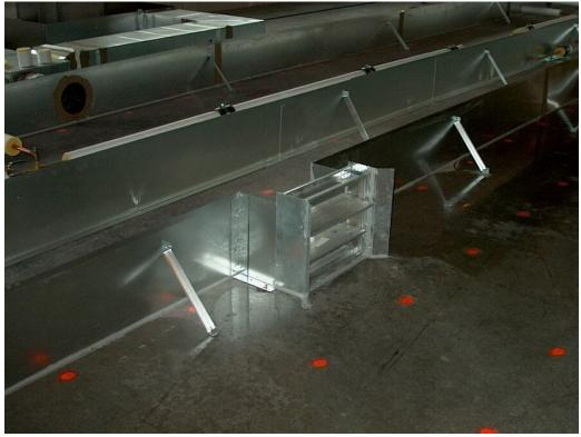
Typical Type A supply air chase way outlet Pic A8
