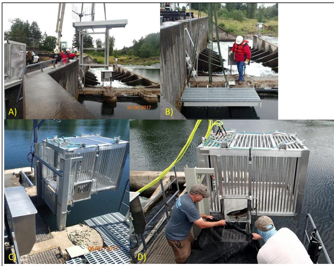
Figure 15. Installation of the Lebanon adult fish trap deck (A & B), photo of the initial trap installation (C) and photo of the pneumatic trap lines and fish capture (D) in 2017 at Lebanon Dam.
