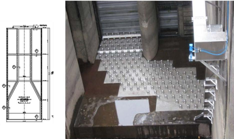
Figure 2. Variable-width entrance weir (line drawing, left) and Bonneville Dam Cascades Island entrance during installation of bollards, Lamprey Passage System (LPS, ascending wall to right in photo), and Half-Duplex PIT antennas (white bars spanning opening near entrance bulk head). The variable-width weir was installed to the entrance slot in spring 2009.
