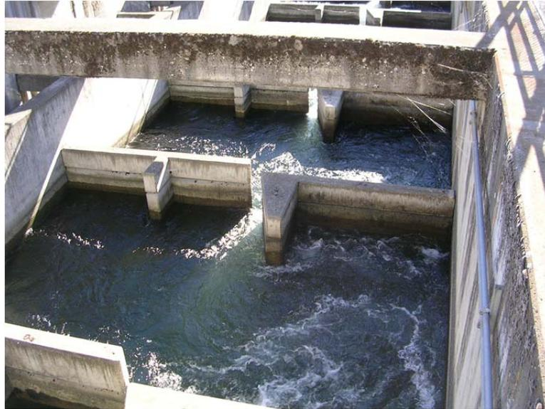
Figure 15: Vertical slot weirs at The Dalles Dam North fishway. Note linear alignment of slots compared to Bonneville Dam serpentine weirs.
