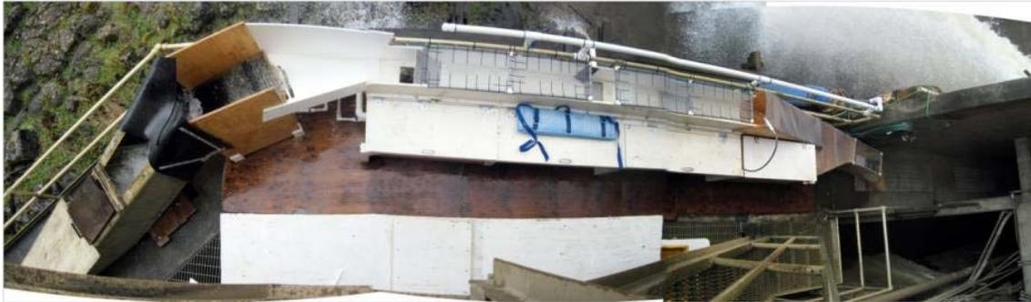
Figure 1. Overhead view of the Denil (left), trap, and ladder return (right) used to collect adult salmon and steelhead at Willamette Falls Dam in 2011-2014.
