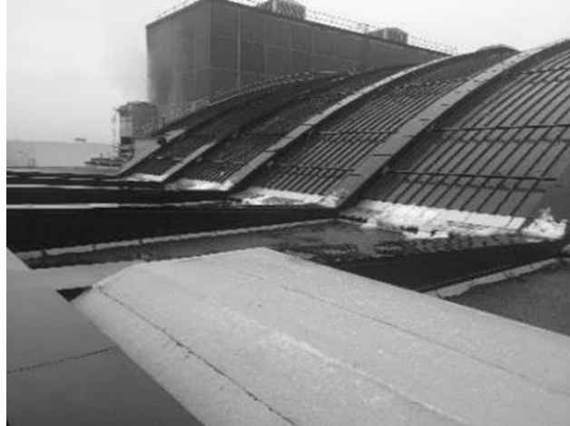
Figure 2: Section of War Memorial roof viewing toward Southwest.
