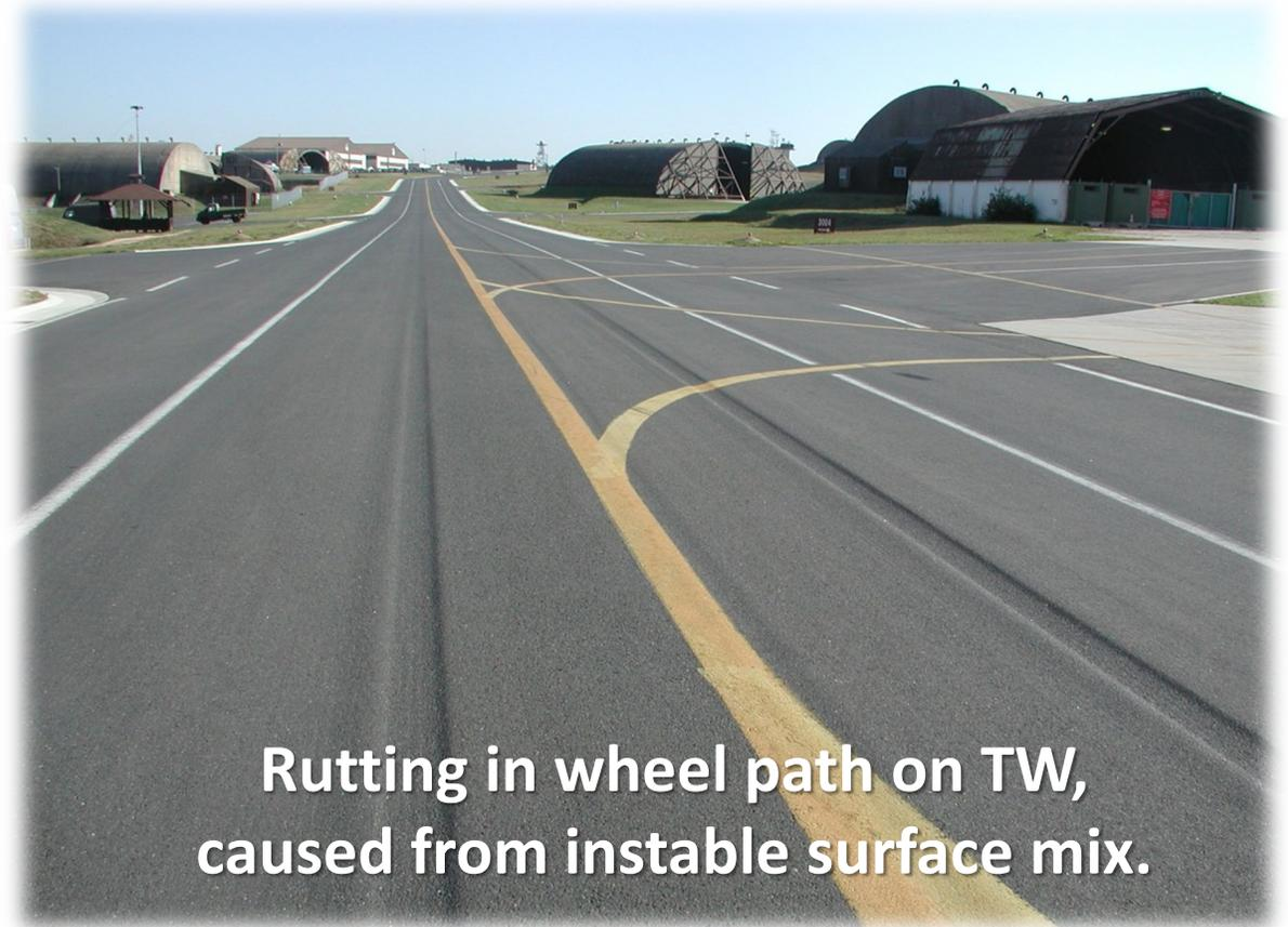
Rutting in wheel path on TW, caused from instable surface mix.
