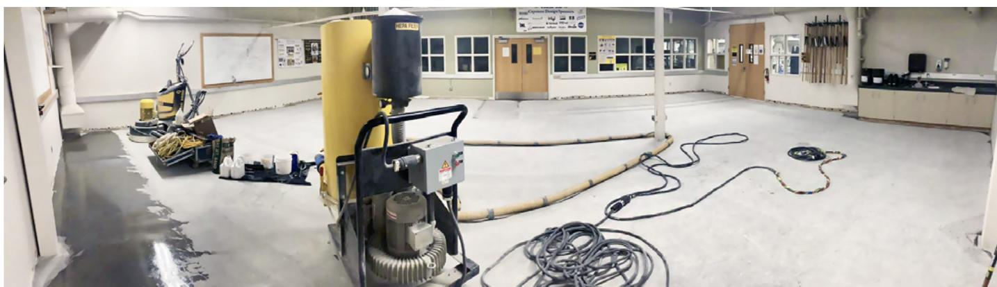
(Above) Phase 1 of the Senior Capstone Design Suite renovation includes cleaning and repolishing of the laboratory floor. Removal and re-arrangement of ceiling ductwork is currently underway. (Below) Phase II will include adding more windows.
