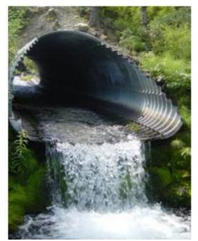
Figure II.10. Poorly designed culverts block upstream fish passage. Photo: Cecil Rich.
