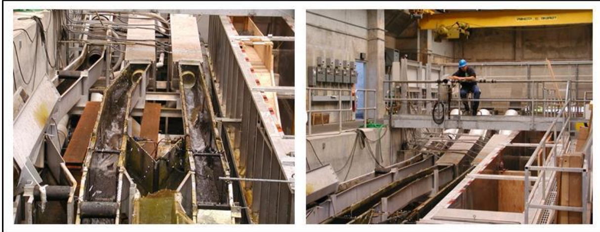
Figure 2. Left: the adult fish facility (AFF) at Bonneville Dam, showing the flumes below the false weir where fish exited the holding pool (behind technician in photo on right). Adult fish were selected for radio-tagging by the by a technician who initiated a pneumatic gate that diverted fish to an anesthetic tank at the base of the chutes (not shown).
