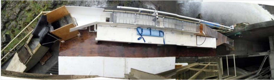
Figure 1. Overhead view of the Denil (left), trap, and ladder return (right) used to collect adult steelhead and Chinook salmon at Willamette Falls Dam in 2011-2013.
