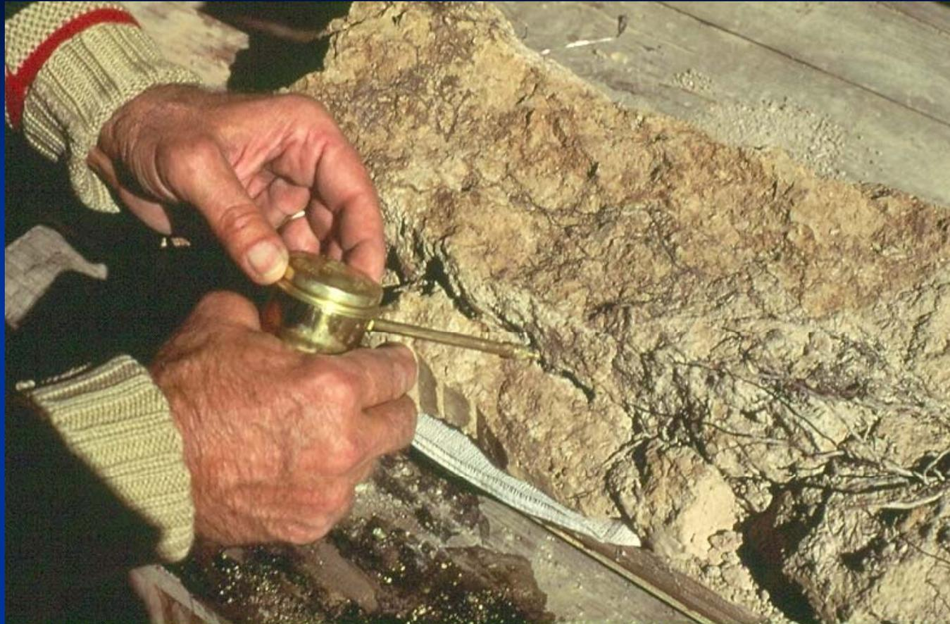
Fill cracks and openings along edges with cellulose acetate.
