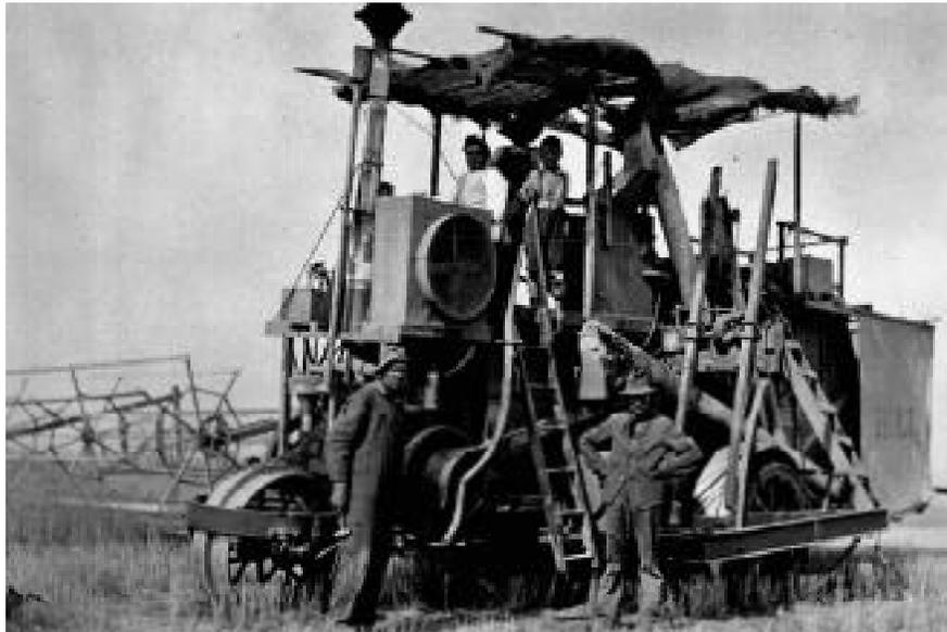
Harvesting grain in 1919 with a converted self-propelled Holt engine.
