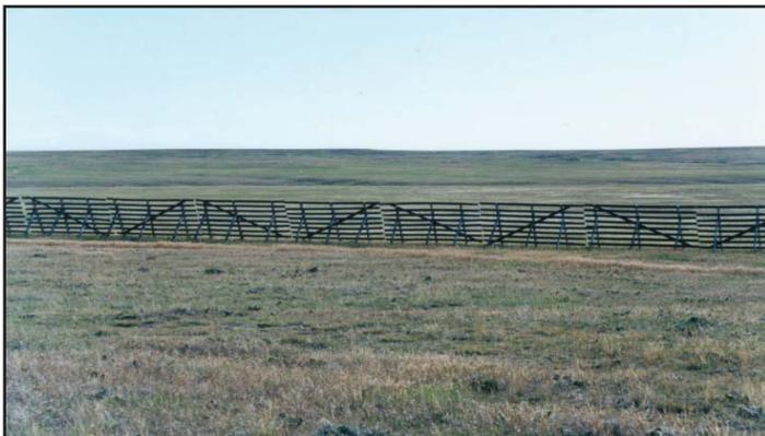
**Figure 1.** Structured barrier used to trap snow.
