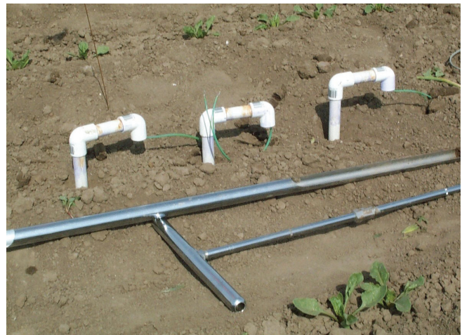
Figure 8. Completed installation of a sensor "station."
