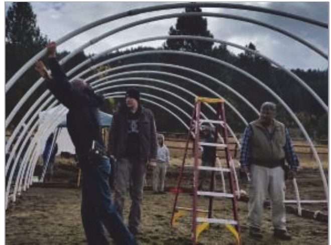
Raise the Hoops program constructed a 26-foot high tunnel in partnership with the Idaho Center for Sustainable Agriculture.
