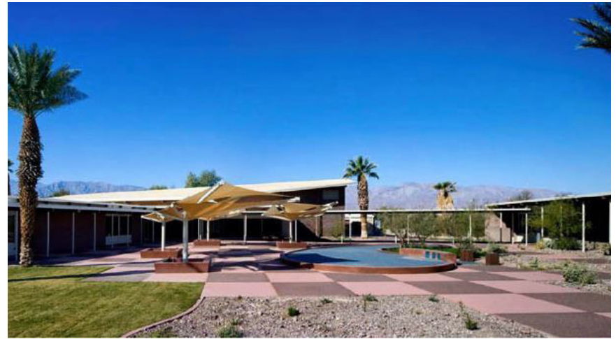
Furnace Creek visitor center complex courtyard. It includes shade structures, a shaded walkway, and a pool for visitors. This image also portrays the balance between lawn and native vegetation.
