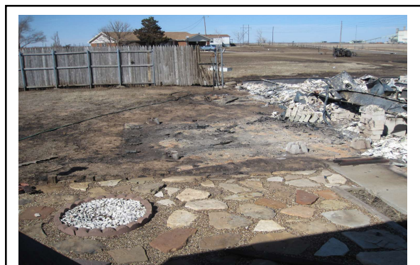
A combustible fence served as a pathway, leading fire right up to this modular home on the Willow Creek South Complex.
