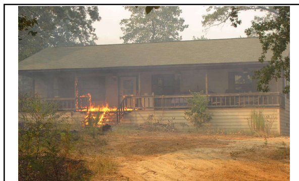
Relatively fire-resistant homes can ignite during low-intensity wildfires if a path of combustible material, such as stairs or support beams, leads the fire up to the home.
