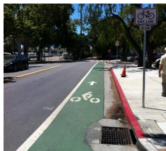
Figure 12. Continuous Colored Pavement Marking for Bike Lane
