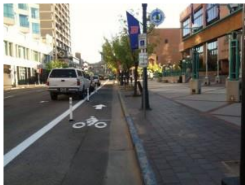
(a) flexible bollards
