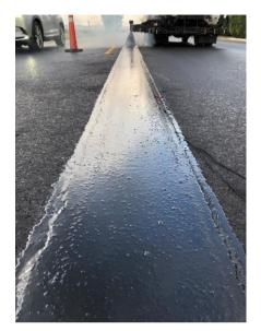
Improving HMA Pavements with a Void Reducing Asphalt Membrane
