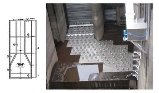
Figure 2. Variable-width entrance weir (line drawing, left) and Bonneville Dam Cascades Island entrance during installation of bollards, Lamprey Passage System (LPS, ascending wall to right in photo), and HD-PIT antennas (white bars spanning opening near entrance bulk head).
