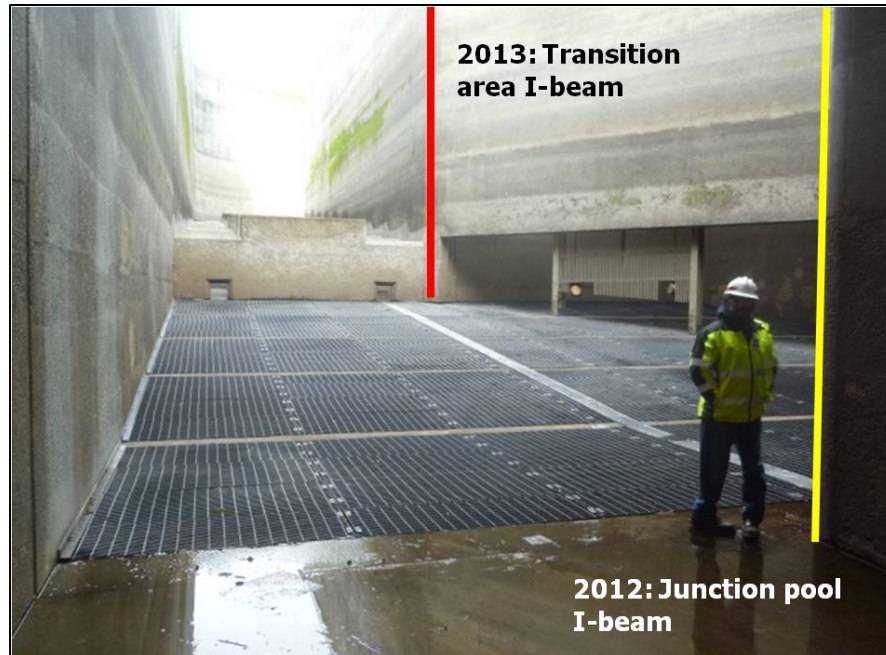
Figure 28. Bonneville Dam junction pool and transition area looking upstream from the NDE collection channel toward Weir 8. The red and yellow lines represent the approximate locations of the I-beams that the DIDSON was deployed onto. DIDSON deployments in the junction pool from 2012 were made on the yellow line in the near-field with the sample volume capturing the area approximately above the square of diffuser grating in the lower left corner of the diffuser grating field. 2013 deployments in the transition area were made on the red line at the overflow weirs.
